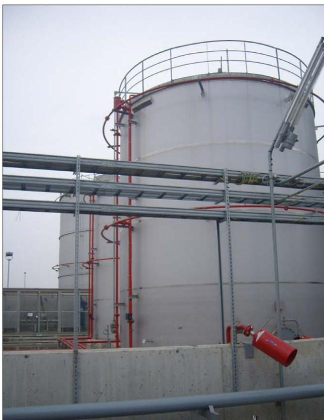
Fig. 2 - Fixed surface system and sprinklers
