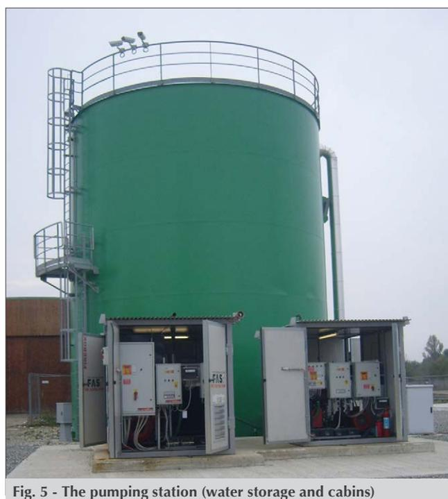
Fig. 5 - The pumping station (water storage and cabins)
