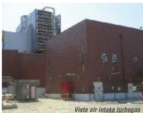
Vista air intake turbogas
