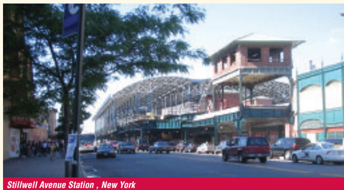
Stillwell Avenue Station , New York
