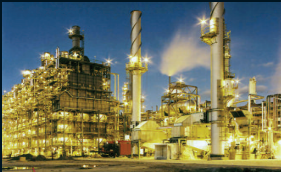
Oil refinery pipelines, Norway
